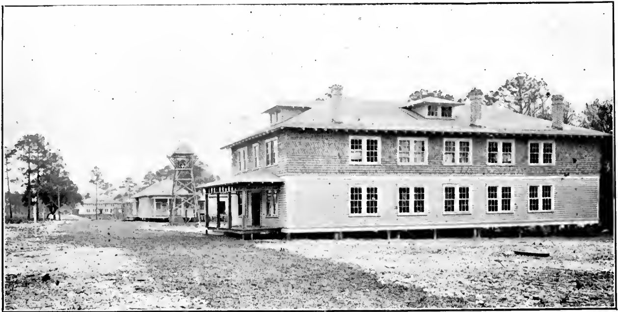
PARTIAL VIEW OF THE NEW HOME OF FLORIDA BAPTIST ACADEMY
